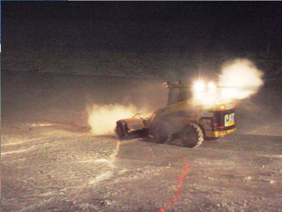
Photo 5: View of Bobcat (equipped with brush), cleaning central key trench area (around station 0+80).
