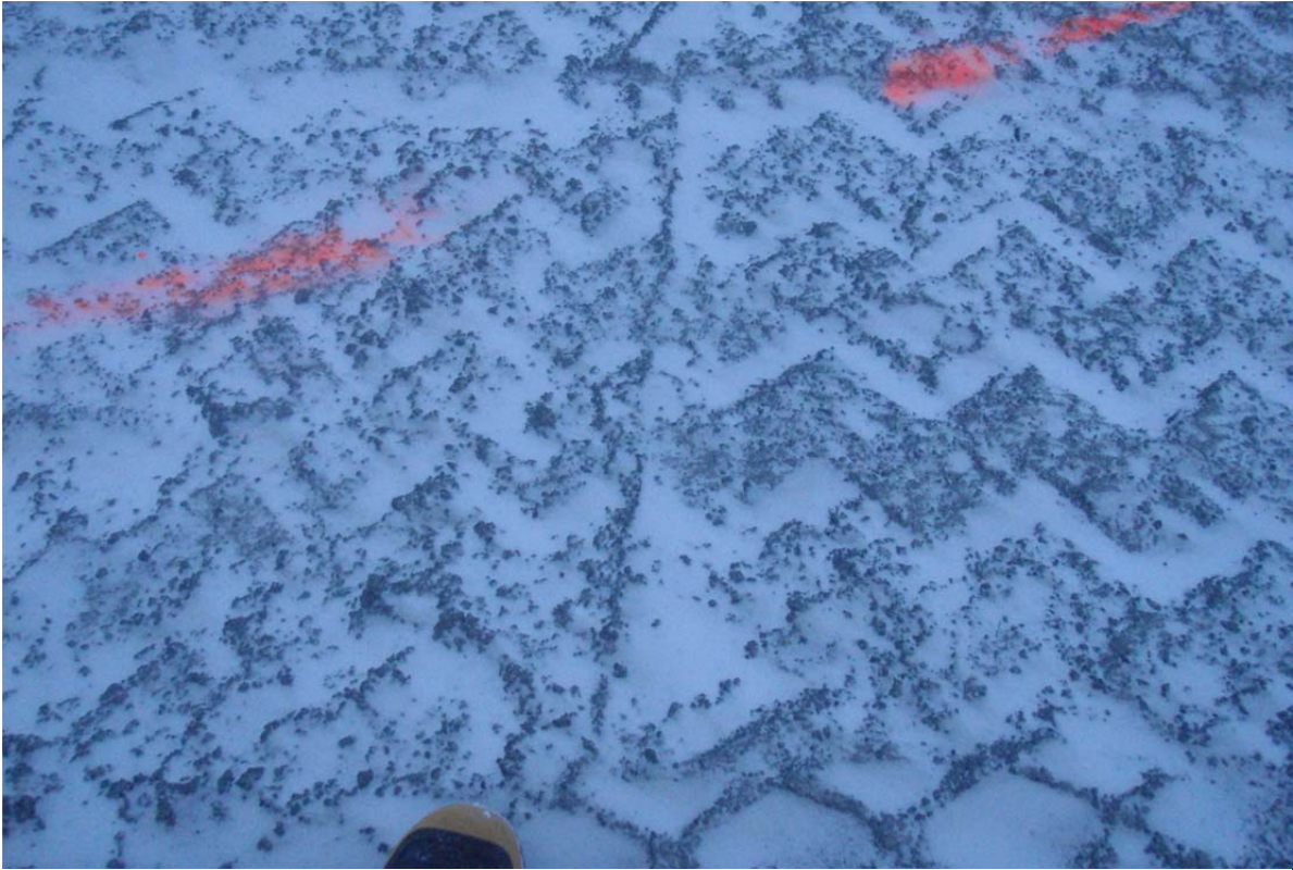
Photo 2: Close up view of Frozen Core Material surface. Note that this material was placed on 2011/01/15. Note the 'zig zag' compactor drum marks on the freezing surface.
