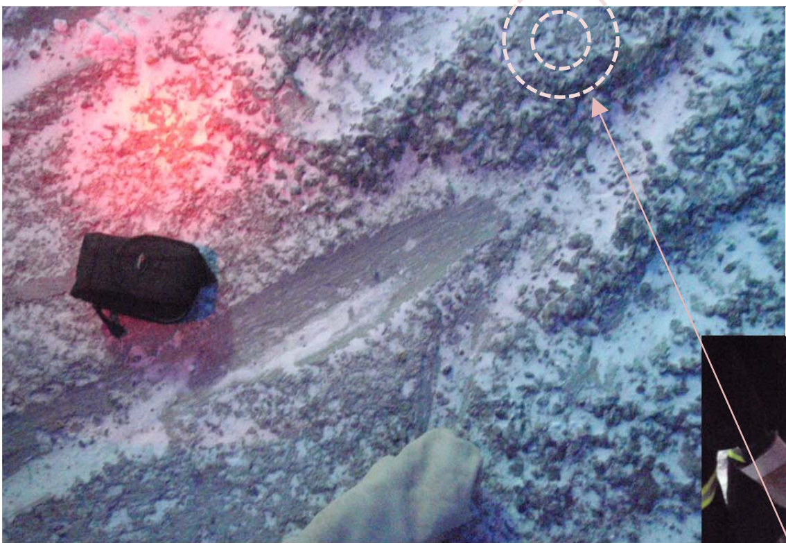
Photo 9: Close up view of cleaning in progress. Note the coarser 5/8" material in relation to the finer core material. The dashed circle shows approximately what the cored location looked like prior to coring. Note: scraping/ cleaning activities were not fully completed around this area at the time of this picture.
