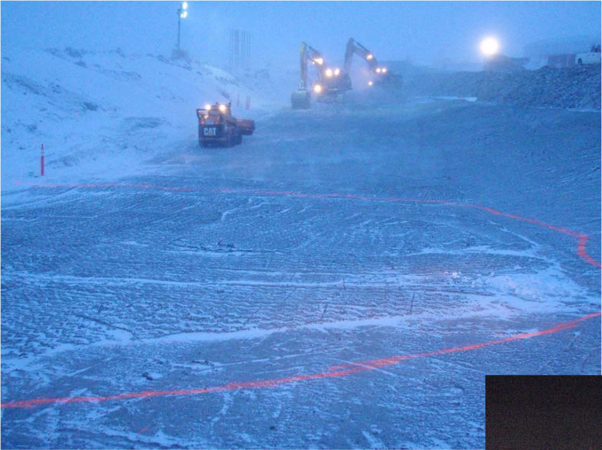
Photo 3: ~NE view of the area where the next center lift is planned to be placed. Note the excavators and bobcat cleaning/ scratching the key trench surface in the background.
