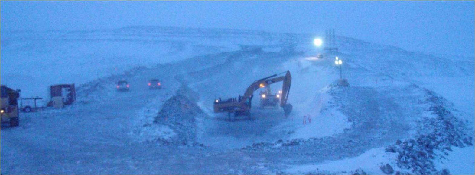
Photo 7: ~ WSW view of construction progress in the key trench.
