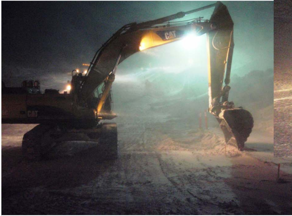
Photo 4: ~W view of the Excavator cleaning snow and 5/8" material in the key trench (around station 1+10)
